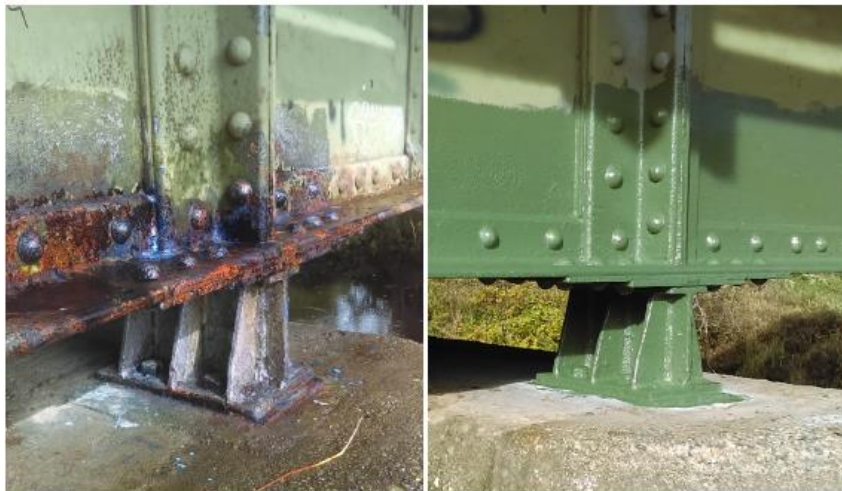
Figure 7. Before bridge maintenance painting (left) and after (right).
